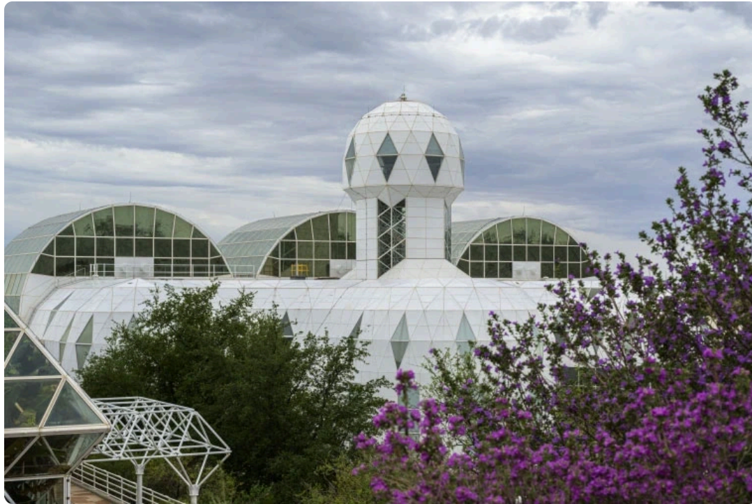
An outside view of the LEO Survey's three experimental hillslopes at Biosphere 2.
